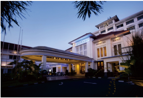
Gambar 2.1 Main entrance Hotel Grand Inna Garuda Yogyakarta Sumber: EHK Hotel Grand Inna Garuda Yogyakarta
